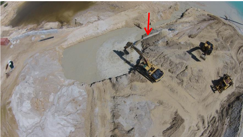
Close up of secondary spoils pit, dredge pipe in operation
