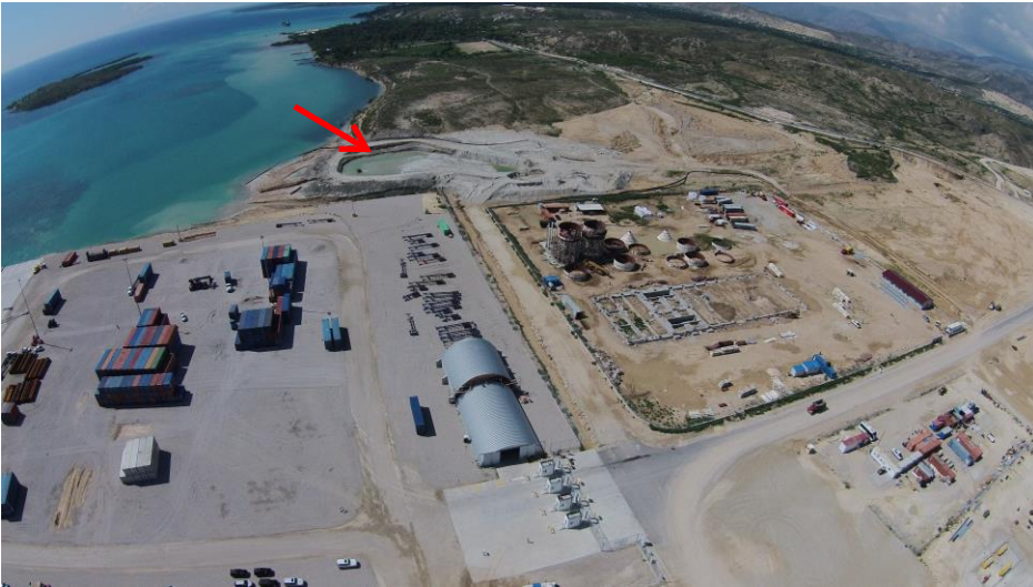
Original spoils pit
